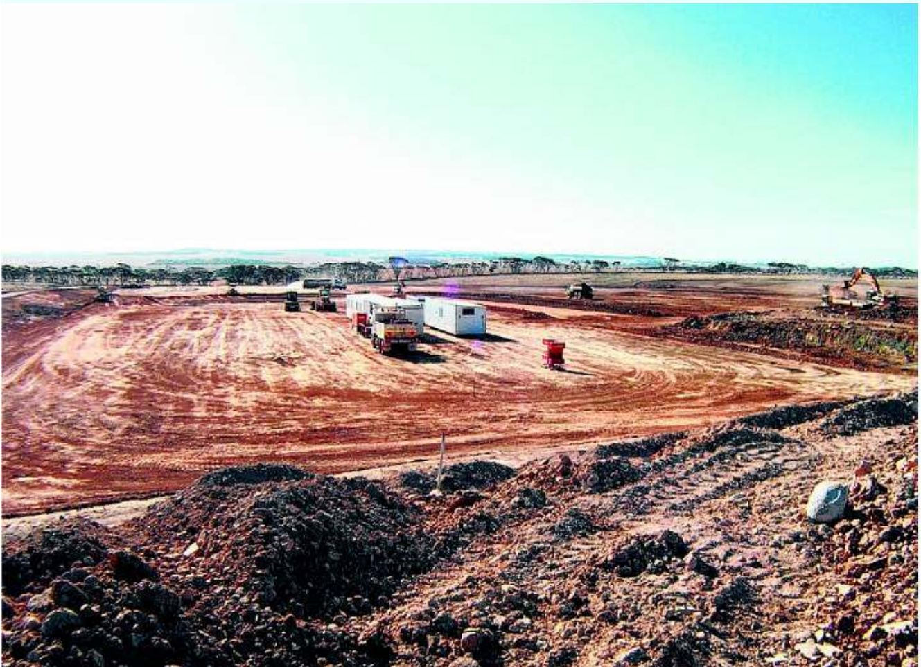
Work has started on Galaxy Resources' Ravensthorpe lithium mine
