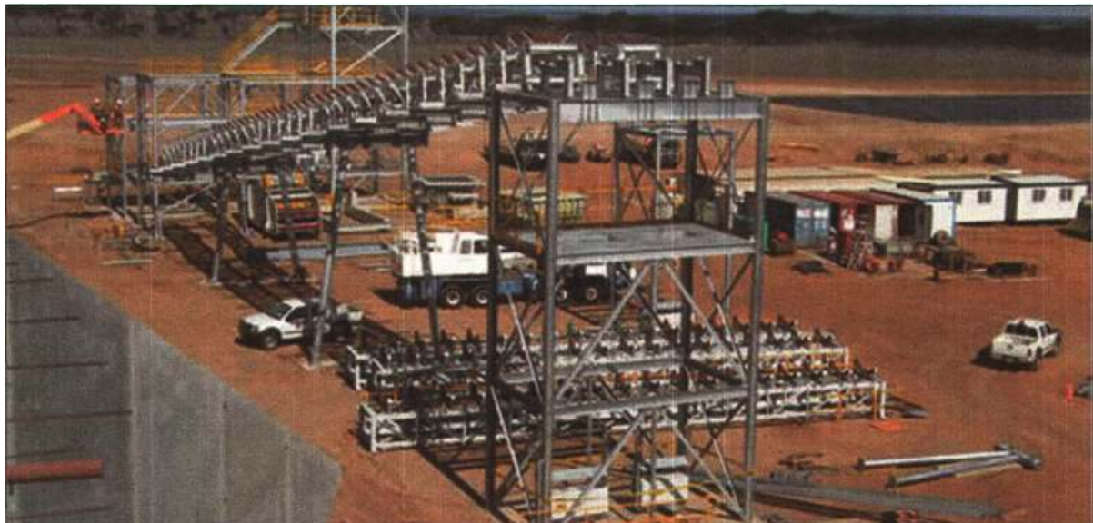
Conveyors from screening plant to secondary crusher
