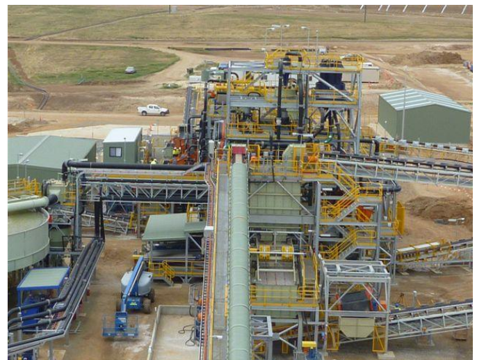
Construction of Mt Cattlin DMS plant
