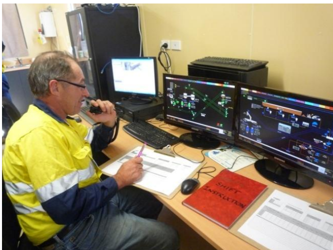
Mt Cattlin control room
