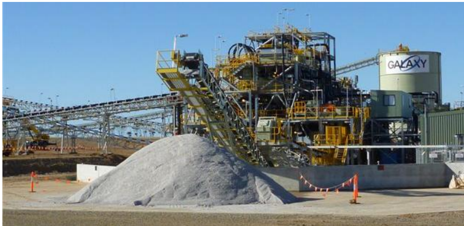
Mt Cattlin concentrator plant
